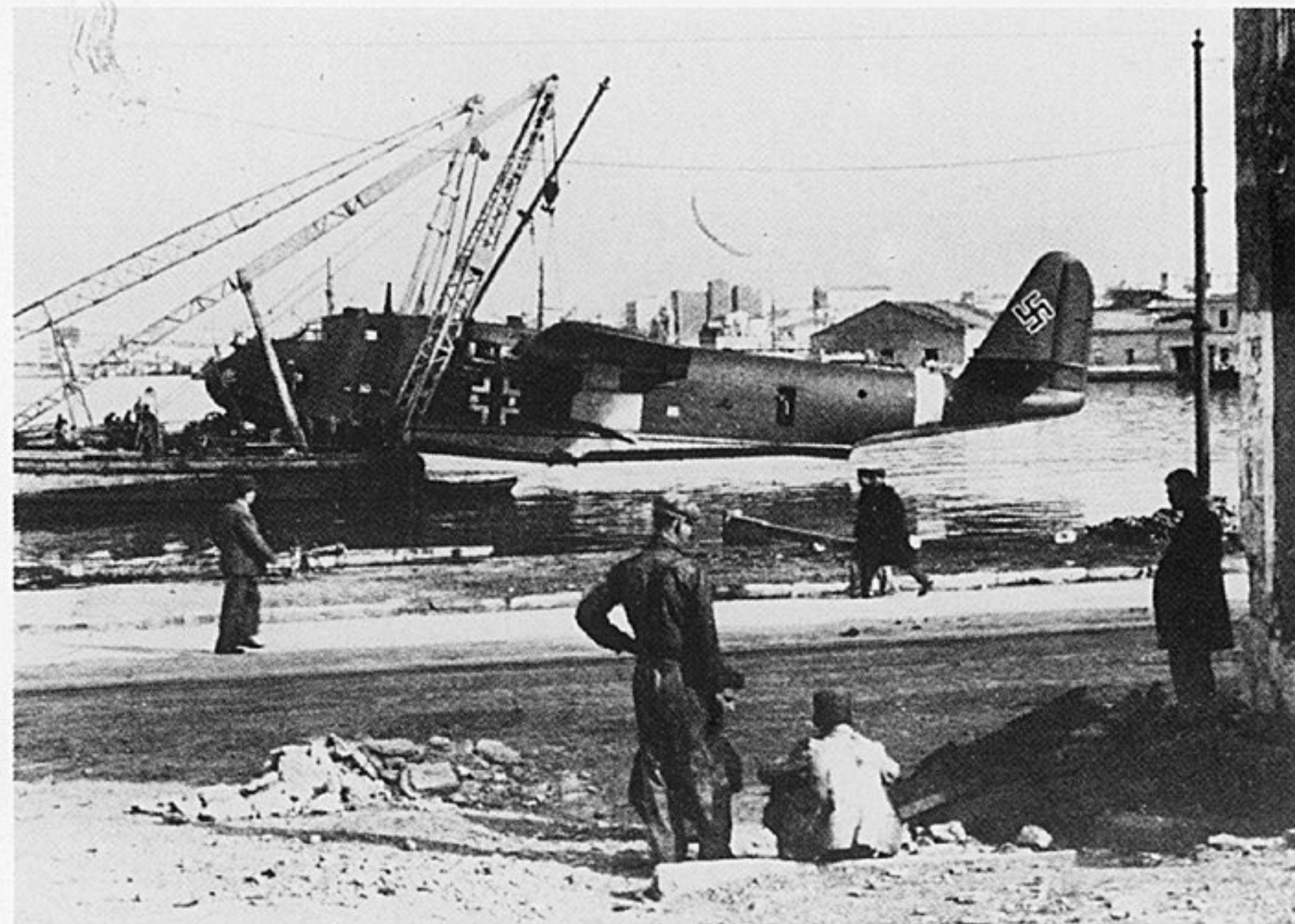
Bv 222 V 2 during repairs on the hull bottom, in Piraeus on 16 December 1941.
